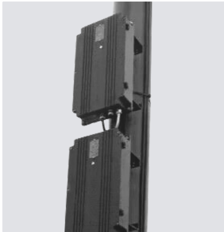
Control Gear fixed on the pole
